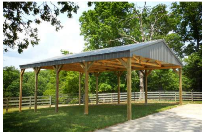
Figure 4.12: Example of open air pole barn. Image Credit:
