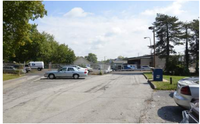
Figure 4.4: Existing entrance into National Road Park (2017).
