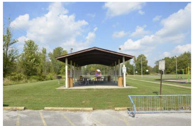
Figure 2.19: No accessible route to picnic shelter at Lions Park (2017).
