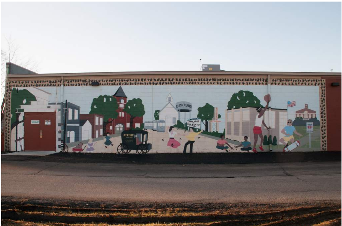
Figure 2.2: Mural along backside of Dollar Tree building facing National Road Park. Image Credit: Town of Cumberland
