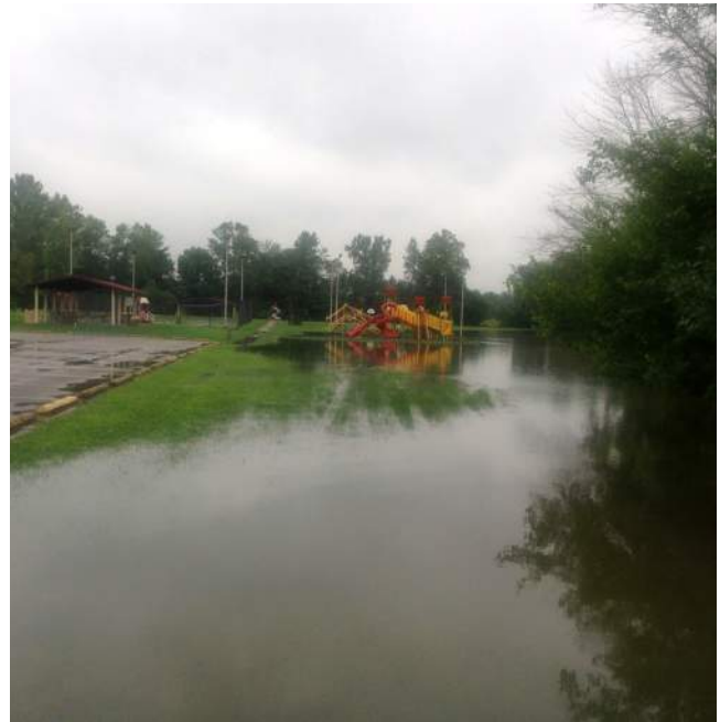
Figure 4.11: Flooding at Lions Park. Image Credit: Town of Cumberland
