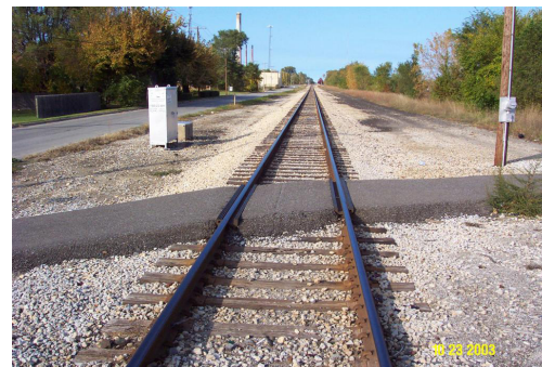
Existing Rubber Panel, Rail Crossing - Amtrak Rail Line Michigan City, Indiana
