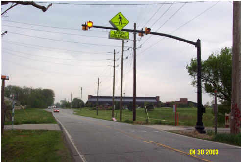
Example of an At-grade Crossing Level 2 - Monon Trail Carmel, Indiana
