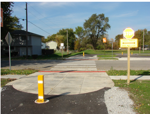
Example of a Concrete Node Entry with Bollard
