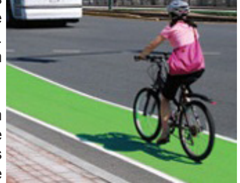
Example of Epoxy Bike Coating on Asphalt
