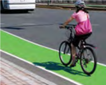
Example of Epoxy Bike Coating on Asphalt
