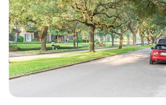
Medians are likely to be the most useful on higher volume, higher speed roads as opposed to lower speed roads. Medians should not replace potentially better solutions such as wider sidewalks, bicycle lanes, buffer strips, and on-street parking depending on the areas that are having problems that need to be addressed. To learn more, **click here**.
