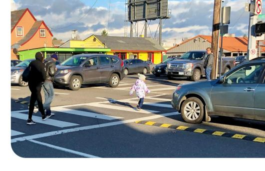
Data collection showed that left turn calming effectively reduced vehicle turning speeds by an average of 13%, with greater reductions observed when "noses" were included in the design. Additionally, the technique nearly eliminated instances of drivers crossing the centerline, which can increase crash risk. Hardened centerlines using rubber bumps proved to be nearly as effective as those using delineator posts while being more cost-effective and easier to maintain.
