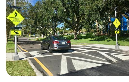
pedestrians. These crosswalks should be installed in areas where there is a significant pattern of pedestrian street crossing (i.e. the middle of a block with development on both sides). Crosswalks can be designed with pavers or other distinctive materials that help define the crosswalk. Speed tables are designed to increase driver awareness of pedestrians, and make drivers slow down more than if they were approaching a speed hump.
